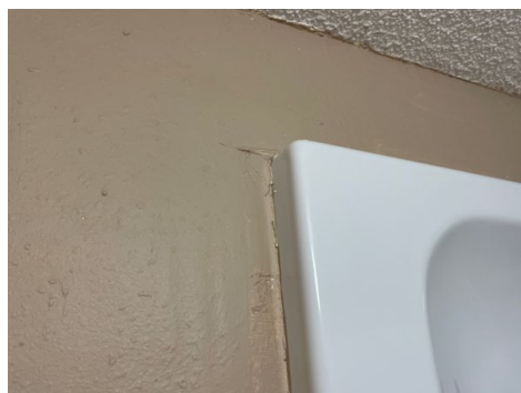
Small drywall patching around shower
