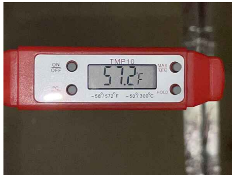
Supply Air Temperature
