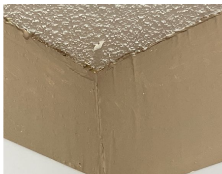
Small drywall patching around shower
