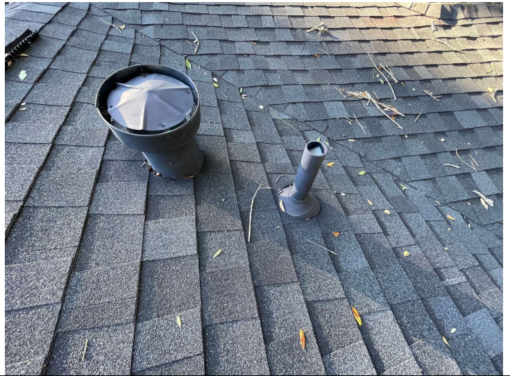
Roof Penetrations (All vents have new boots)
