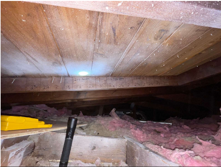
Roof Deck Thickness (Sheathing in 1" x 6" Tongue and Groove Lumber)
