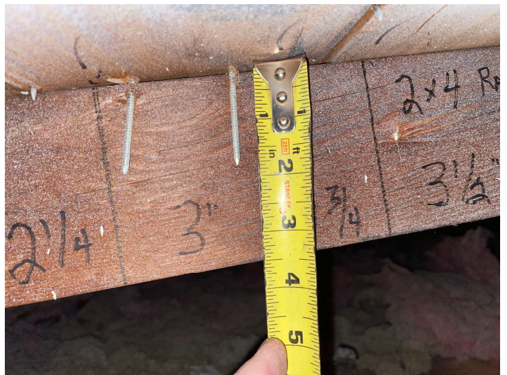
Roof Deck Fastener Size (Appears to be 8D Nails)
