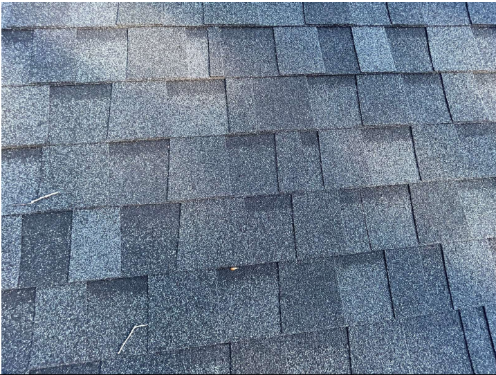
Roof Covering (Architectural Asphalt Shingles)
